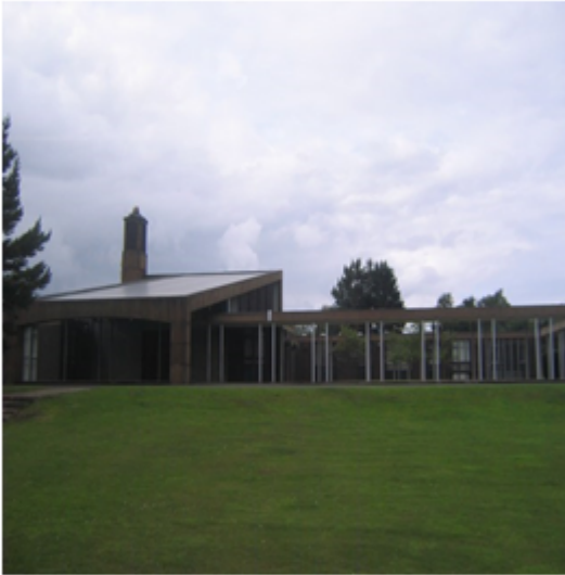
Crematorium general view
